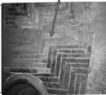
Figure 9. The tessellated bricks on Brunelleschi's Duomo (Florence, Italy) and equivalent structure of conch shell.
